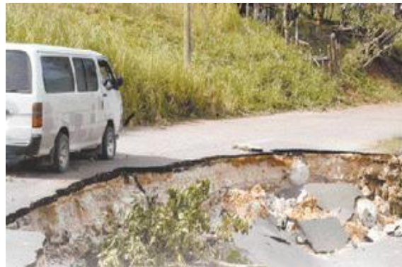
Van navigating around section of road been damage by landslide
