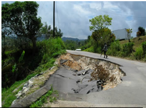
The retaining wall gave way resulting in the road been damaged
